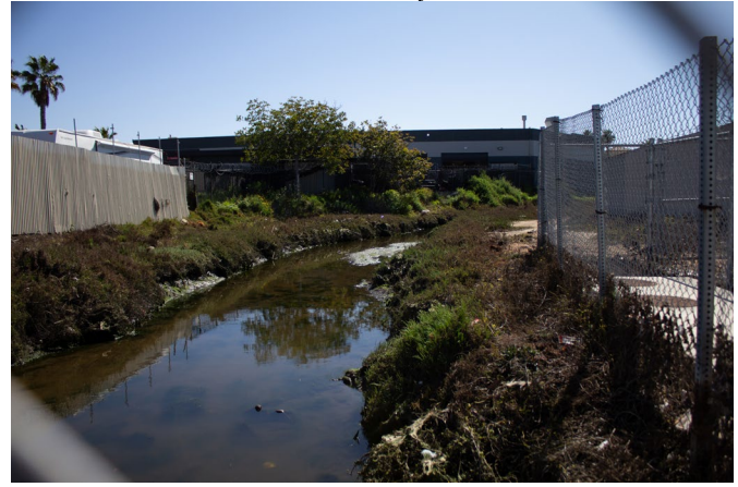
View of Paradise Creek adjacent to the Welding Shop on West 18th Street in National City. The creek is prone to flooding due to king tides and heavy rain events.
