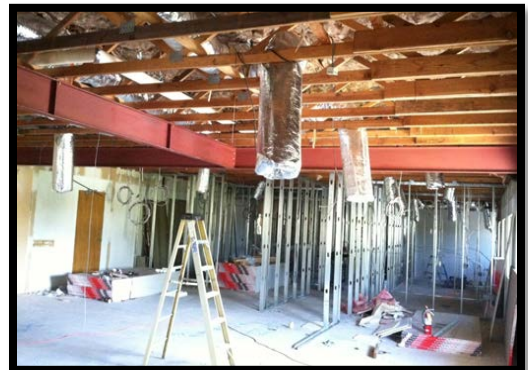
Work began on Interwork Institute's new space
