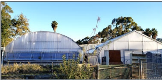
6361 Alvarado Ct Greenhouse – Exterior
